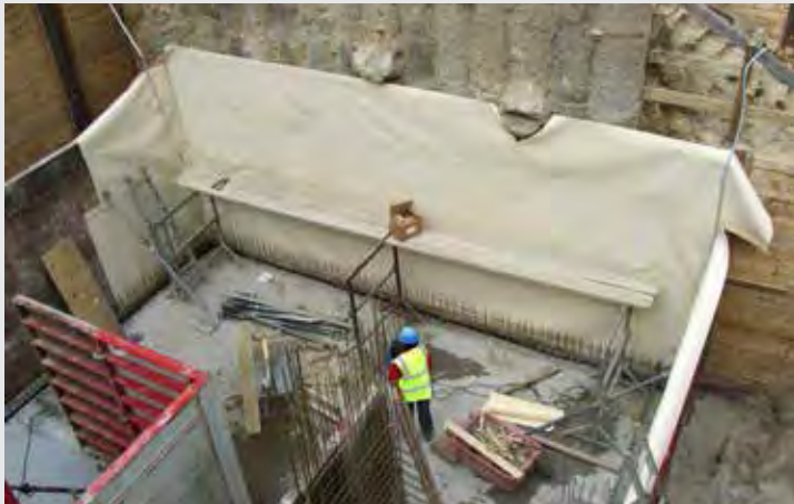
Walls, single- or double-faced formwork
