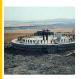
During this windmill installation, one of the biggest challenges was the wind! The grouting had to be completed before 10:00 am, when the winds started to pick up. Pouring of Sikadur VPC structural grout started at 7:00 and was completed by 8:30. The windmill base needed to be strong enough to provide the required structural stability by 10:00, for the tower installation. Sikadur Injection Gel Fast Set was applied to create perfect bedding. Once everything was levelled in place, Sikadur VPC
