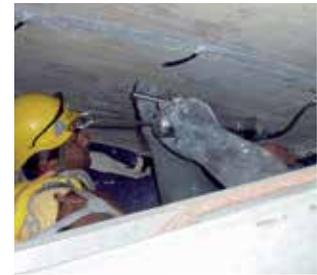
Remedial solutions for cracks and joints: Sika® Injection, Sikaflex®, Sikadur® Combiflex System
