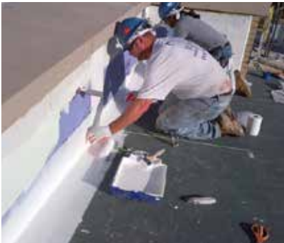
Step 4 - DETAILING/FLASHING
