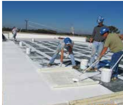
Step 5 - MEMBRANE APPLICATION
