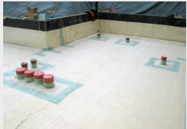
Finished internal jointing detail
