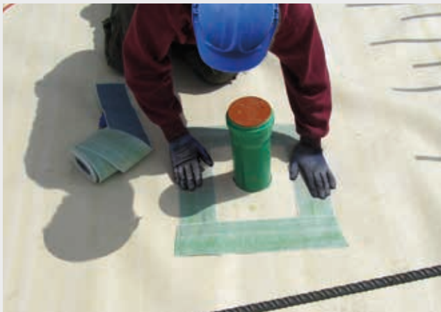
Internal jointing detail with SikaProof® Tape-150
