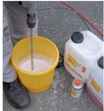
Mixing of an acrylic injection resin
