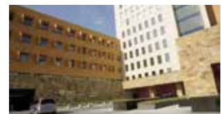
Centro Médico Zambrano Helion, Monterrey (Mexico): Use of Sikagard® protective and hygienic wall coatings.
