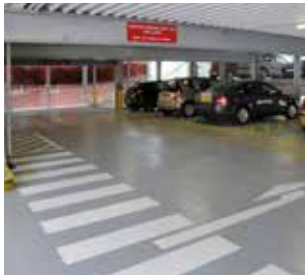
Sikalastic® parking deck membranes and Sikafloor® coatings for pedestrian areas (including safety markings paint).
