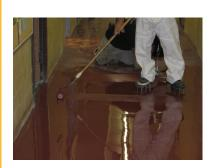
Once this stage was completed, Sikafloor® 261<sup>CA</sup> - Systems 5 and 6 were installed. The first step involved applying a self-levelling top coat, followed by a coat of Sikafloor® 2003 to create a slip-resistant finish. The final stage consisted of filling the control joints with Loadflex®, a load-bearing, self-levelling, control-joint filler.
