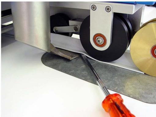
Using a flat metal plate for starting welding at seams and ribs. This will allow for some adjustment of alignment and for the automatic to achieve proper speed before making contact with the PVC overlap.
