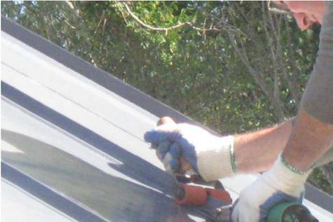
At starts and stops as well as in areas that are not suitable for machine welding, hand welding is required. A “two headed” silicone roller which can be made with parts from two single rollers, facilitates the process.
