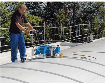
The rib guide attachment is just that, a guide. Chalk lines are still required as the guide is only intended as an aid to keeping the ribs equally spaced.
