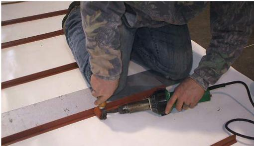
Another method for keeping ribs straight is to use a simple straight edge made of sheet metal as shown here.
