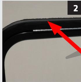
**WARNING:** Applying the primer using masking tape to delimit the application area will not prevent leakage through the masking tape.
