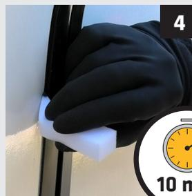
**4** With the pad, apply a thin, uniform coat of **Sika® Primer-207** along the application surface area and in the joint. Allow to dry for ten (10) minutes.
