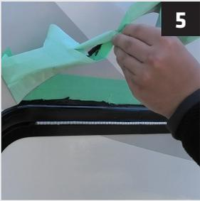
5 Immediately after application, carefully remove the masking tape.
