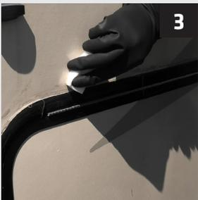
**3** Use a **Sika® PowerClean Aid** pad with a small amount of water and clean to ensure that the application surface is clean, sound, dry and free of any contaminants (dust, oil, grease, etc.).
