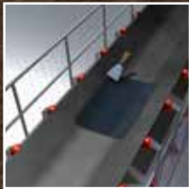
Conveyor belt repair and bonding
