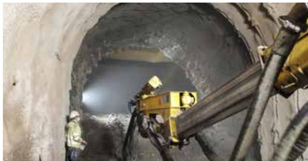
SikaFiber® Force synthetic macro-fibres were added to the sprayed concrete to increase the ductility of the concrete lining. Fibre-reinforced sprayed concrete of this kind produces a more efficient and cost-effective excavation support.
