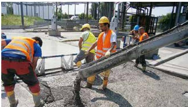
SikaFiber® Force synthetic macro-fibres were used in combination with the German 'White-topping' method for repairing the slabs in an oil harbor in Stuttgart. The fibres were used to improve the fatigue behavior of the new concrete topping.
