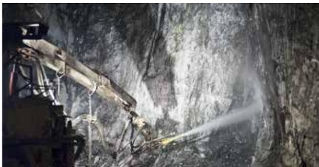
In this mining project, SikaFiber® Force synthetic macro-fibres were used for the sprayed concrete, mainly as the excavation support. Their selection and use ensured an efficient, cost-effective and safe work flow as driving advanced.
