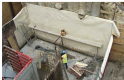
Walls, single or double face formwork
