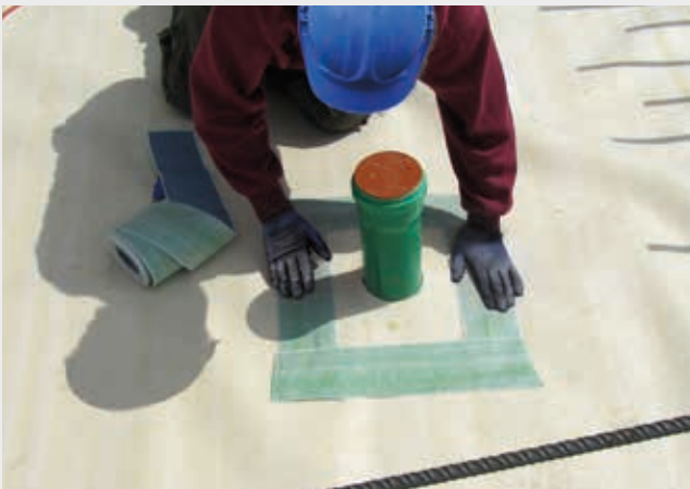
Internal jointing detail with SikaProof® Tape-150
