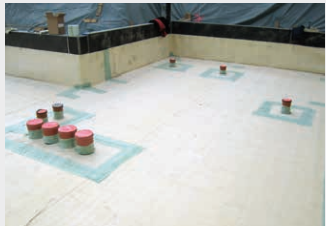
Finished internal jointing detail
