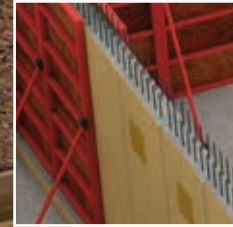
Walls, double formwork
