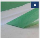
Immediately after application, carefully remove the masking tape.
