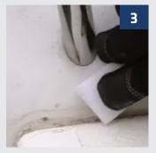
Use a **Sika® PowerClean Aid** pad with a small amount of water and clean to ensure that the application surface is clean, sound, dry and free of any contaminants (dust, oil, grease, etc.).
