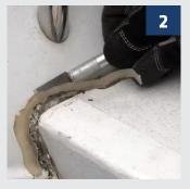
Remove existing sealant with a spatula or scraper and remove residue with a clean cloth.
