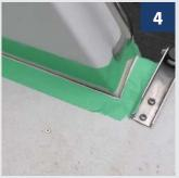
For ease of application, we suggest delimiting the application area with masking tape to prevent preparation products and sealant from being inadvertently applied to glass or paint<sup>1</sup>.
