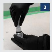
With the pad, apply a thin, uniform coat of **Sika® MultiPrimer Marine** along the application surface area and in the joint. Allow to dry for 30 minutes.
