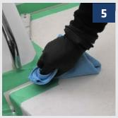
Using a dry cloth or a Sika® PowerClean Aid pad, apply Sika® Aktivator-205 on the application area to ensure better adherence for priming. Allow to dry for 10 minutes.
