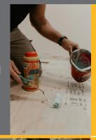
The use of a primer such as Sika® Level-01 Primer<sup>CA</sup> is recommended prior to the application of the self-levelling compound on concrete or cementitious floors. When treating wood substrates, use Sika® Level-O3 Primer<sup>CA</sup>. Apply primer by brush or roller and allow to become translucent before pouring the underlayment.
