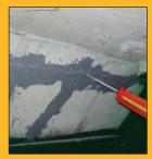
CRACK INJECTION RESINS Sikadur® SikaFix®
