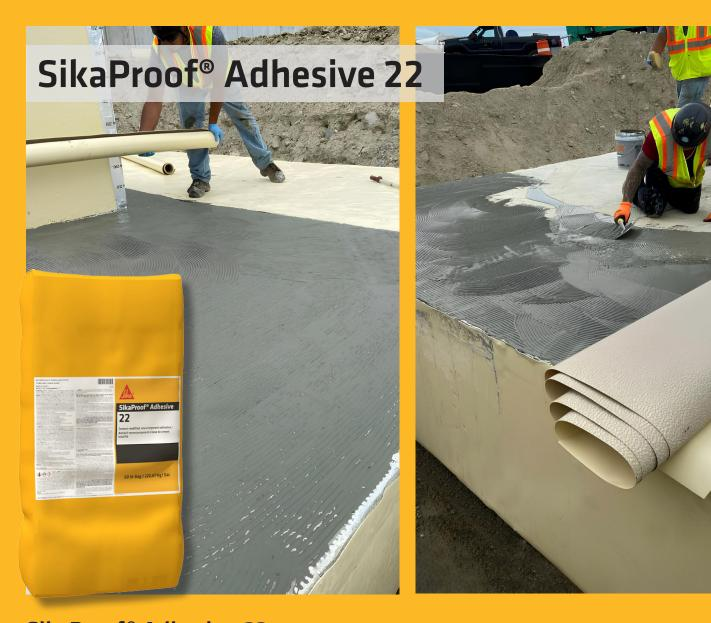
**SikaProof® Adhesive-22** is a single-component, thixotropic cement-based adhesive designed to bond the SikaProof® A+ membrane to both young and fully cured concrete surfaces.
