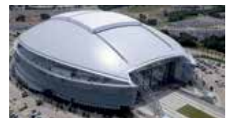
Cowboys Stadium, Dallas (USA): Sika provided flooring, joint sealing, roofing solutions.
