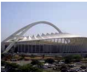
The Moses Mabhida Stadium (South Africa): Sika provided joint sealing, concrete protection and grouting solutions.
