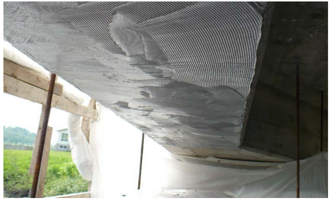
Figure 1: Example of the application of a resinous component
