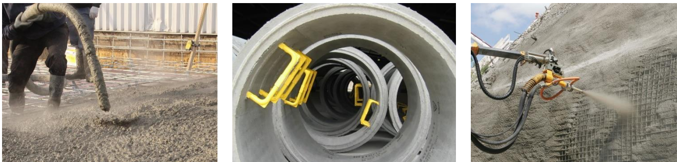
Figure 1: Applications for concrete admixtures (from left to right: air entrainer, dry cast and set accelerator)
