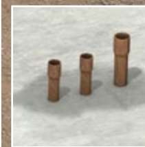
Leaking Penetrations i.e. Pipe Penetrations
