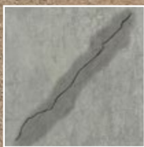
Leaking Cracks
