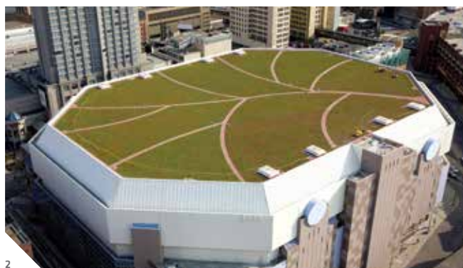
2 Target Center – Minneapolis, Minnesota
