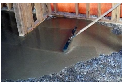
Figure 1: Examples of applications of cementitious components on-site
