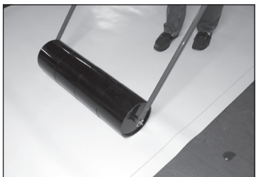
Rolling membrane with a 45 kg (100 lb) roller
