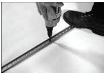
Installing Sarnafasteners
