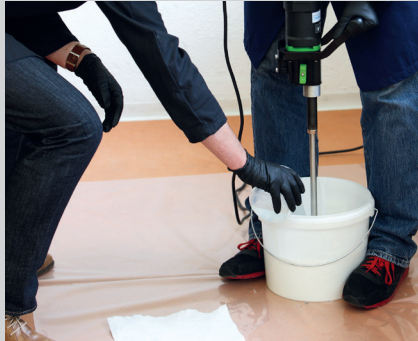
Manual mixing of 2-part Sikasil® GS 687 with cone agitator
