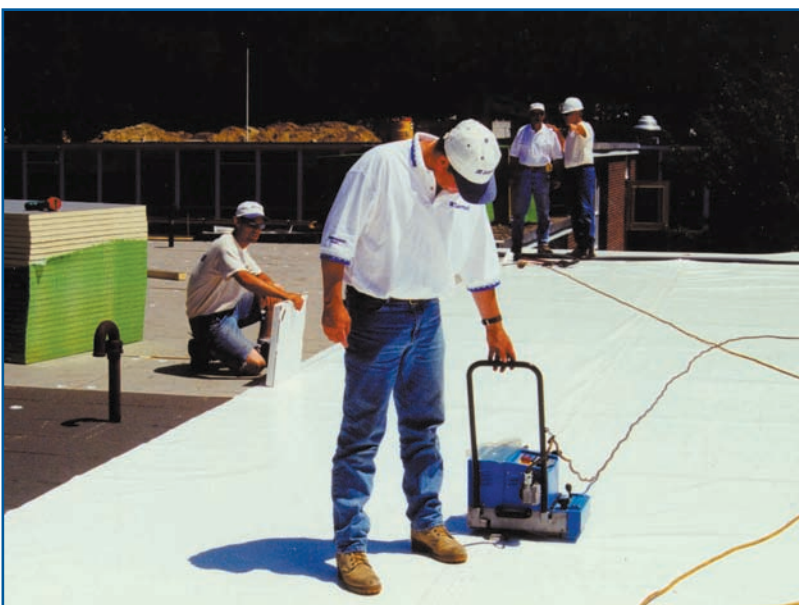
A significant advantage of thermoplastic membrane is the ability to hot-air weld the seams.
