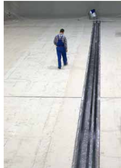
The longest post-tensioned CFRP-plates ever installed
