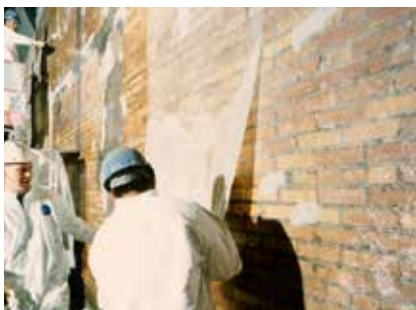
SEISMIC UPGRADING /EARTHQUAKE DAMAGE REPAIR
