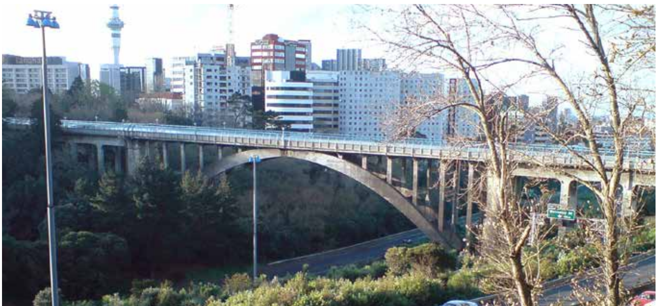
Grafton Bridge, Auckland, New Zealand
