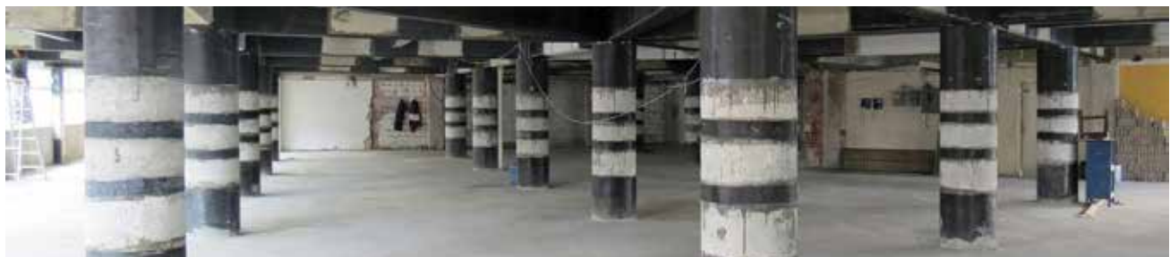
Beams and collums strenghtened with SikaWrap®
