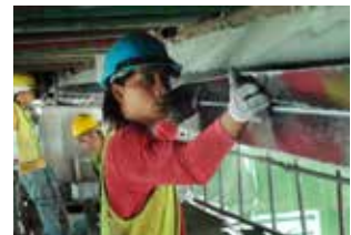
Installation CarboDur®
