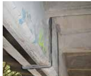
Sika CarboDur® strips and CarboShear L plates bonded to the concrete structure.
