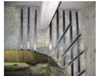
Sika CarboDur® strips and CarboShear L plates bonded to the concrete structure.
