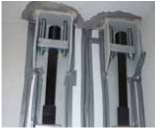
Anchorage of Sika® CarboStress System
