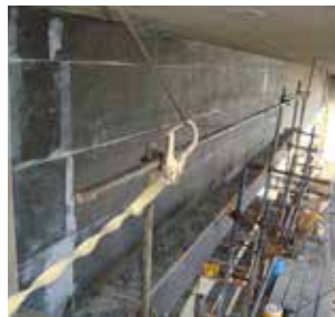
Strengthening with SikaWrap®
