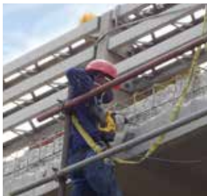
Substrate preparation
