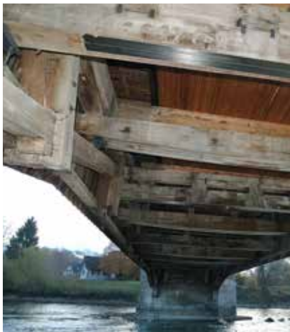
CarboDur® strengthened crossbeam
