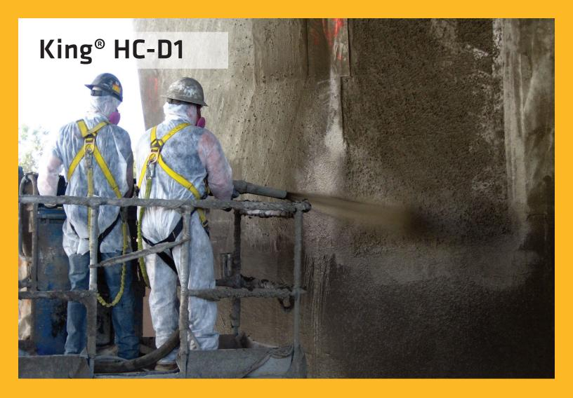
**King® HC-D1** is a shotcrete mix for dry process application. King® HC-D1 is a pre-mixed, factory bagged material for optimum quality and formulated to be compatible with existing concrete substrates, provide very high resistance to cracking and achieve durable repairs over time.
