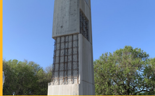
CONCRETE REPAIR & PROTECTION
