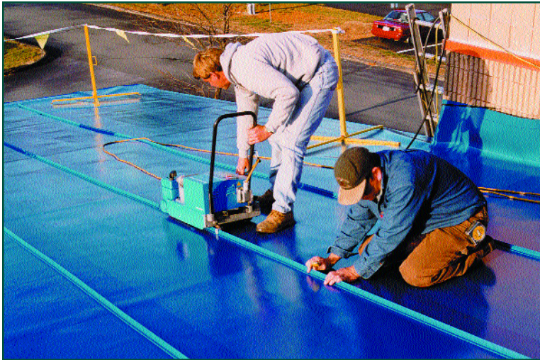
Welding rib in place.
