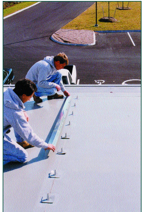
Post and rib installation.
