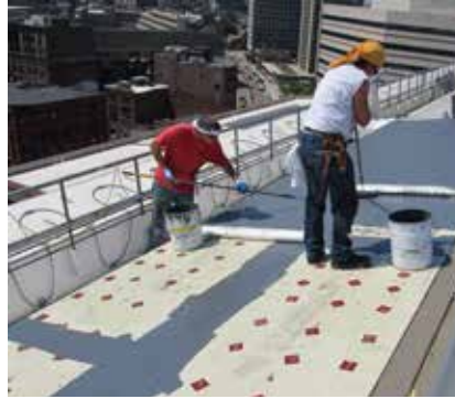
Step 2 - INSULATION/COVER BOARD (As specified)
