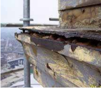
Step 1 - SUBSTRATE PREPARATION
