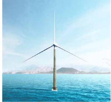
For the precast elements of the tower the following concrete was used: Concrete type: HAC 60-AC-E2/12/3C+E Type of cement: I 52.5 and 32.5 Sika Admixture: Sika ViscoCrete® V-70, Sikament®-230 and SikaTard®-930
