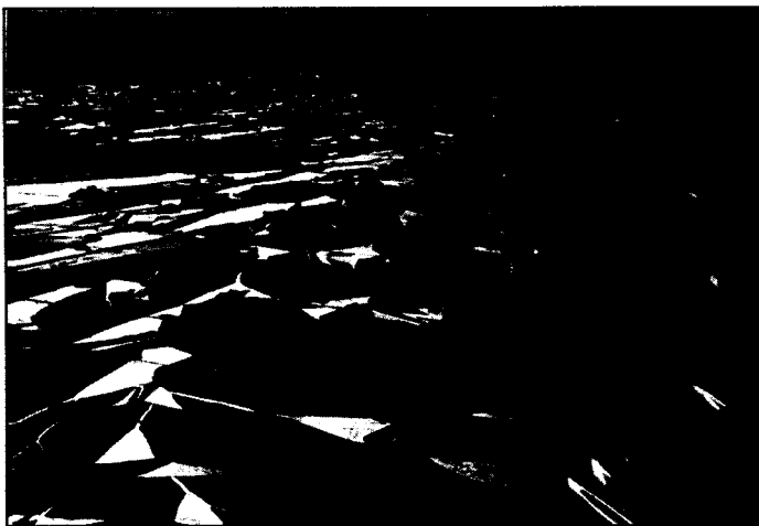
Figure 5. Shatter failure, mechanically attached, nonreinforced membrane.
