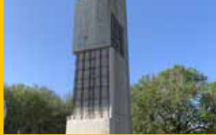
CONCRETE REPAIR & PROTECTION
