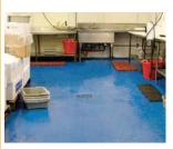
The floors of a high profile fish and seafood supplier to luxury hotels and restaurants were rapidly deteriorating. The existing paint was peeling off the floor causing water to creep under the concrete surface and was creating a damp and slippery environment. The surface of the loading areas was also worn due to high traffic forklift use and the floors of a recent expansion also needed to be coated.
