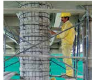
Sika® MonoTop®, Sika® Top® and SikaRepair®: Cementitious mortars for concrete repairs.
