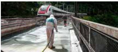
Chärstelenbach Railway Bridge, Amsteg (Switzerland): Sprayable waterproofing membrane on the bridge deck.
