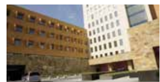
Centro Médico Zambrano Helion, Monterrey (Mexico): Use of Sikagard® protective and hygienic wall coatings.
