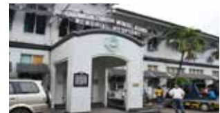
Locsin Montelibano Memorial Hospital (Philippines): Restoration work on a historic building using Sika® Carbodur® structural strengthening systems.
