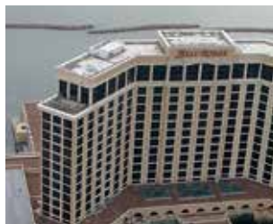
The MGM Beau Rivage, Biloxi (USA): Sika® Sarnafil® roofing system installed on the top of this 29storey-high resort hotel and casino.
