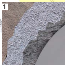
1 First Shotcrete lining
