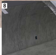
8 Secondary Concrete Lining
