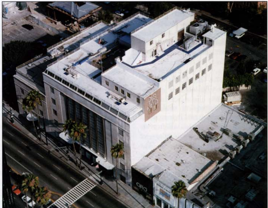
A bird's eye view of a Saks Fifth Avenue rooftop.
