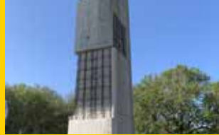
CONCRETE REPAIR & PROTECTION
