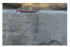
SikaSwell®-A profiles are a range of high performance swellable waterstops for construction joints and pipe or steelwork penetrations in concrete
